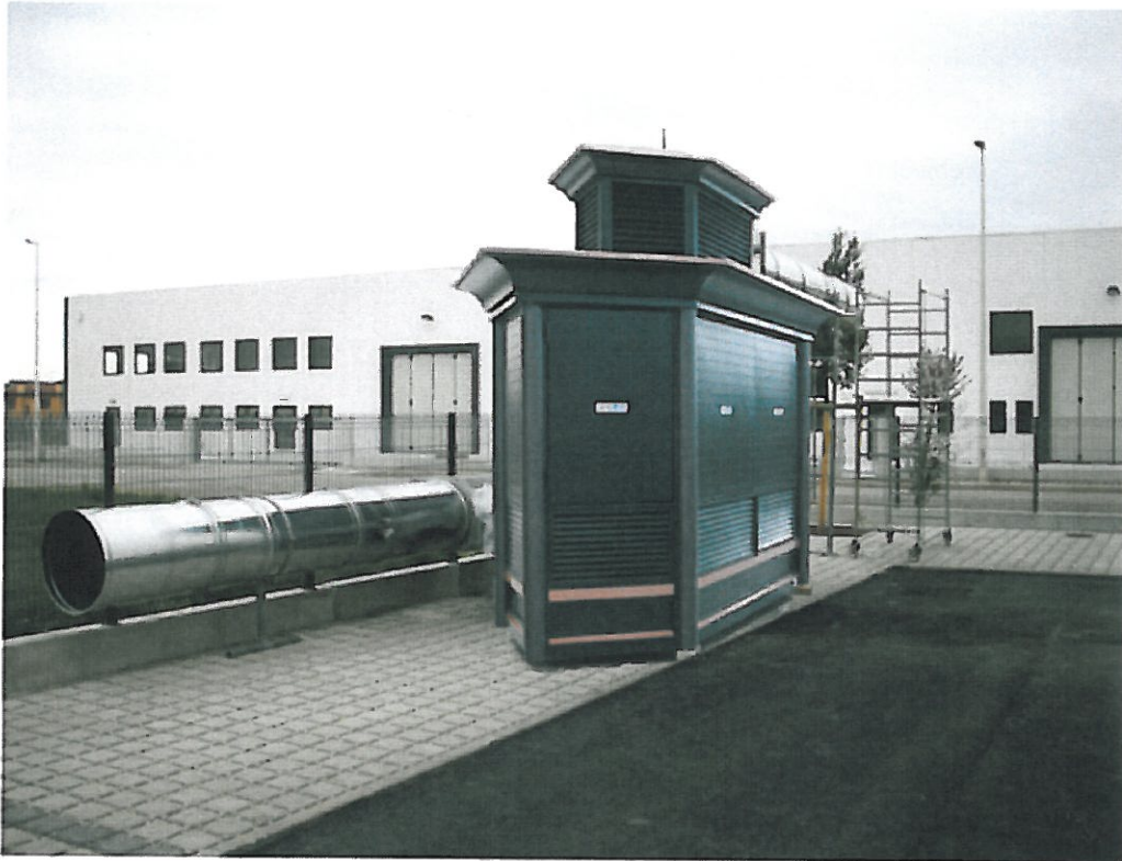
Picture 1: filtration system with the tubes for the sampling
